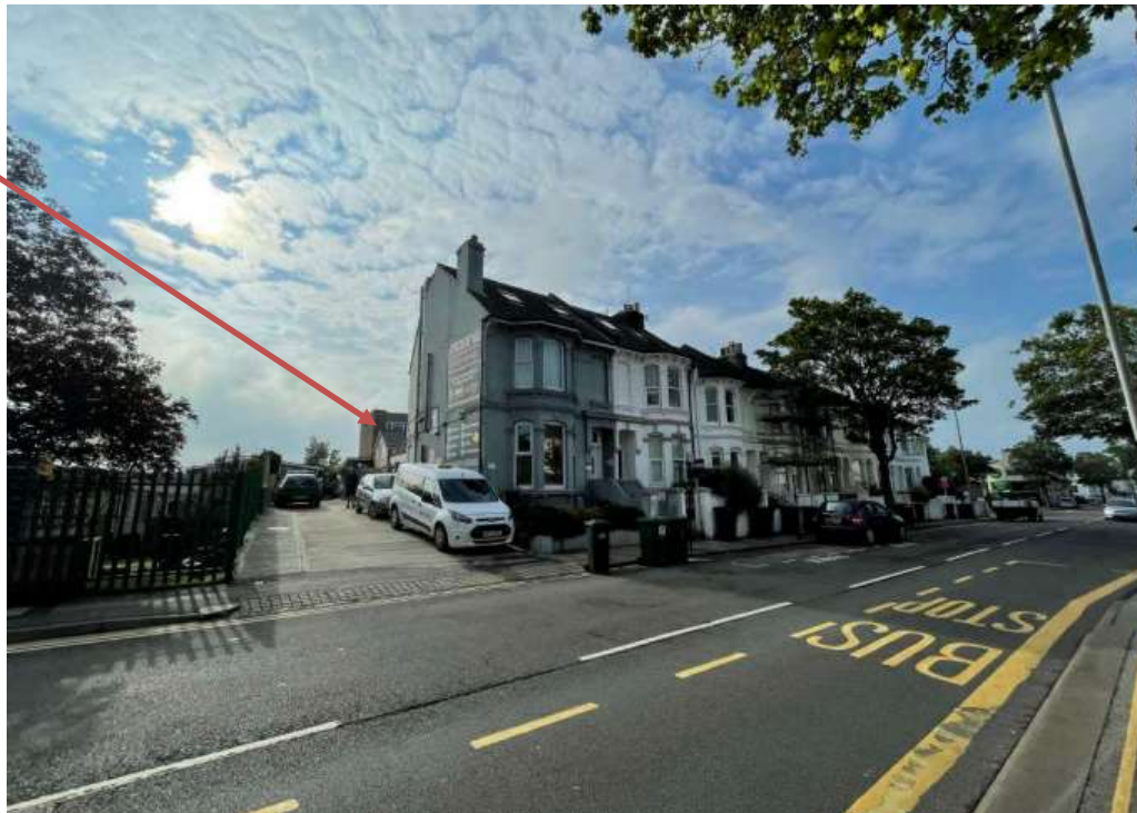
Photo taken from outside No.152 Ditchling Road looking East.
